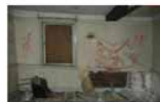
west window wall
