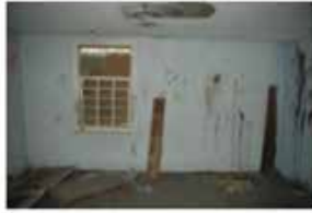
east (window) wall
