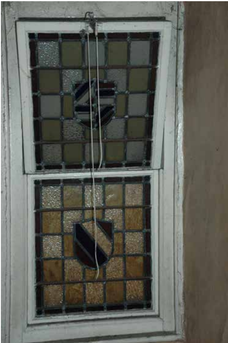
multi-paned staircase window to east wall
