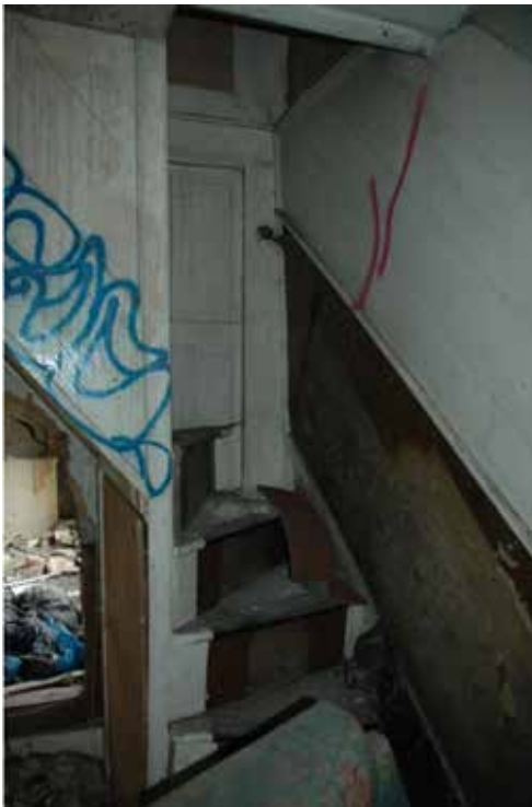
winders and side planking
