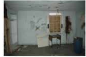
west (window) wall
