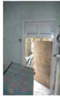
doorway to rear lobby
